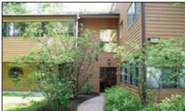
166 Bunn Drive, Princeton NJ • Available: 2,609 SF, Contiguous • 1,139 SF - Suite 106, 1,469 SF - Suite 109 • (CAM Includes All Utilities) • Ideal for Professional Office, Medical/Chiropractic • Parking 4/1,000 SF Covered Spaces • 11,000 SF Building on 5.61 AC • Near Route 1 & Downtown Princeton
