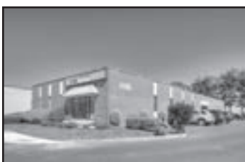
2500 Brunswick Pike (Rte. 1), Lawrence Twp. 789 SF Office/Medical • For Lease Immediately Available Conv. Access to Rt 1 & I-295
